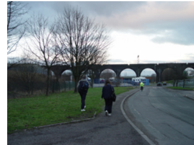
Figure 11.3.6 - Elevated railway viaduct
